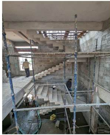
Scaffolding erected for upper-level access; staircase structure being finalized with ongoing interior work.
