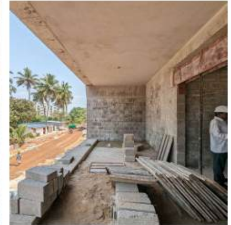
Ongoing block masonry work on the upper floor balcony with material stacking; site supervisor inspecting progress and alignment.
