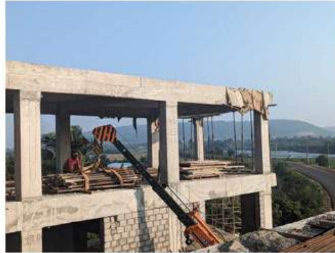
Site overview showing multiple villas under construction; RCC structure and masonry progressing in parallel.
