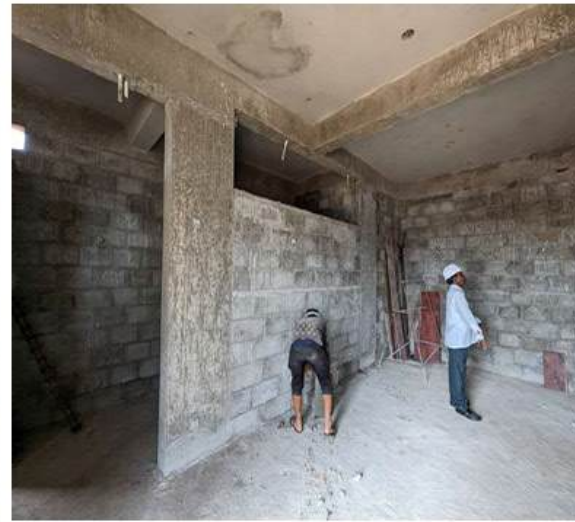
Block masonry work in progress with supervision; internal partition walls being aligned and built.
