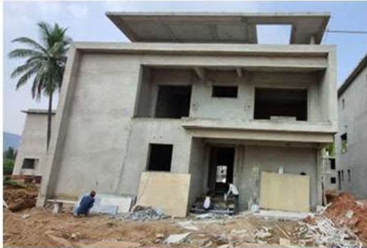
Plastering completed; structure fully defined with balconies and windows ready for fittings.
