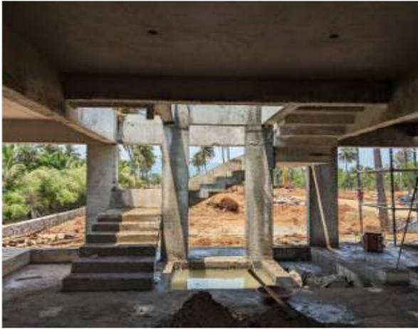
Staircase and slab completed; space opens to the landscape, showing ground-level formwork cleanup.
