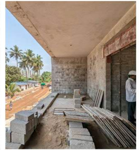
Ongoing block masonry work on the upper floor balcony with material stacking; site supervisor inspecting progress and alignment.
