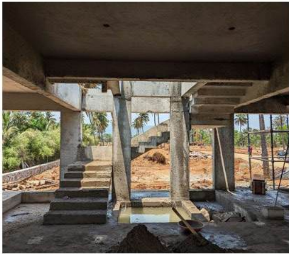
Staircase and slab completed; space opens to the landscape, showing ground-level formwork cleanup.
