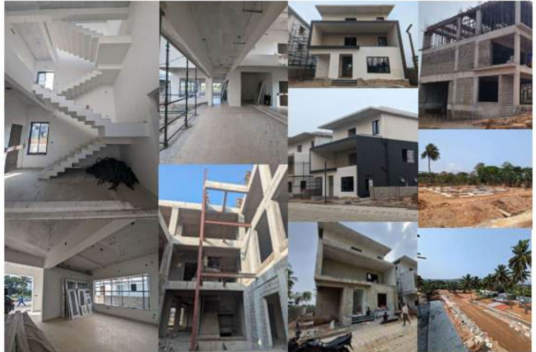
Site overview showing multiple villas under construction; RCC structure and masonry progressing in parallel.
