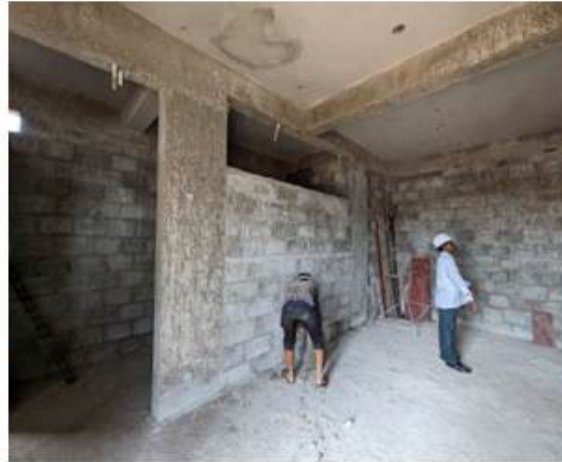
Block masonry work in progress with supervision; internal partition walls being aligned and built.
